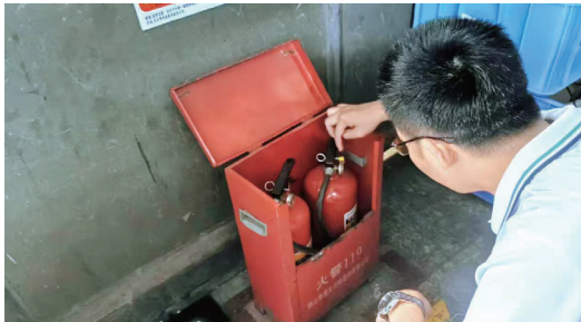
•On-site safety hazard inspection•
