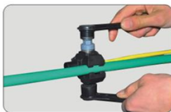
5. The nut will be twisted off when tighten to a certain constant torque. As shown.
